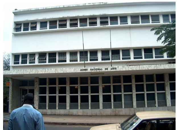
Figure 1. The National Museum of Art in Maputo, Mozambique: front view
