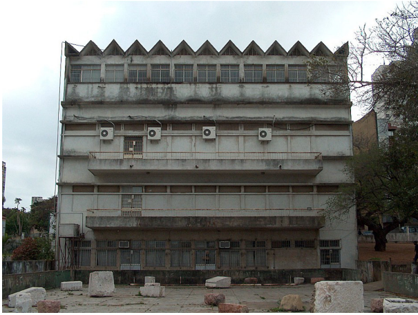
Figure 2. Rear view of the museum showing air conditioners on the first floor and dehumidifiers in the basement
