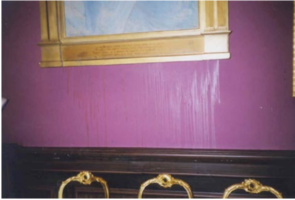
Figure 3. Condensed moisture running down the wall from behind one of several paintings at the Renwick Gallery of the Smithsonian Institution in Washington, D.C. (Photograph courtesy of Ehrenkrantz, Eckstut & Kuhn, Architects)
