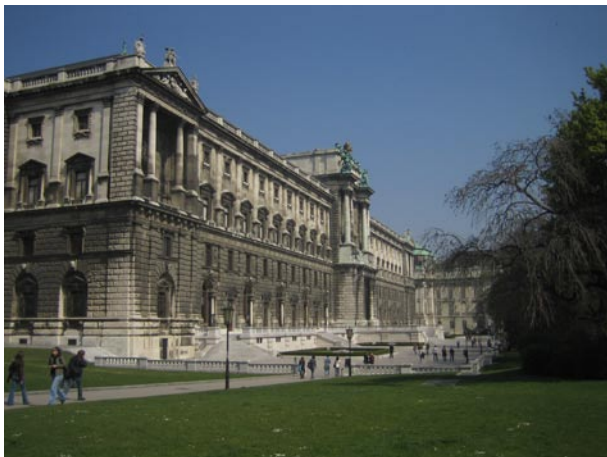
Figure 1. The Collection of Antique Musical Instruments (SAM) is located on the second floor of the Neue Burg. Its 22 windows face the south-east.
