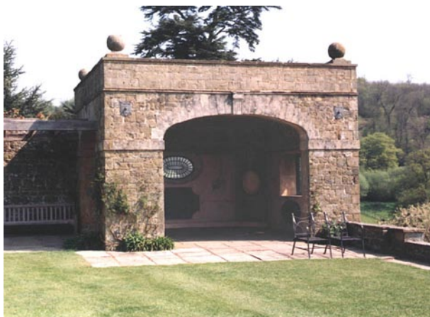
Figure 1. External view of the Marlborough Pavilion from the south
