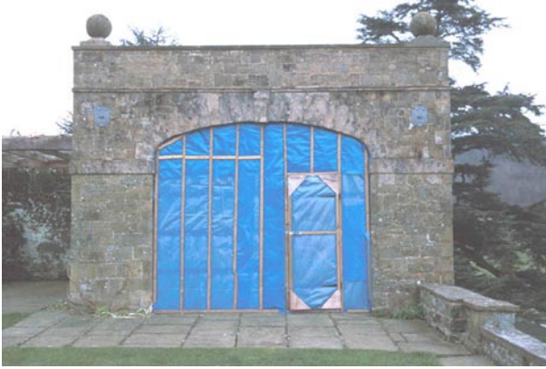
Figure 8. External view of the Pavilion with the initial plastic-covered enclosure
