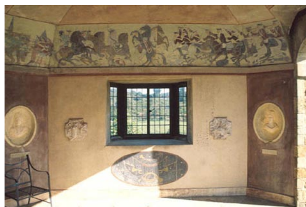
Figure 2. View of the Pavilion's interior before treatment
