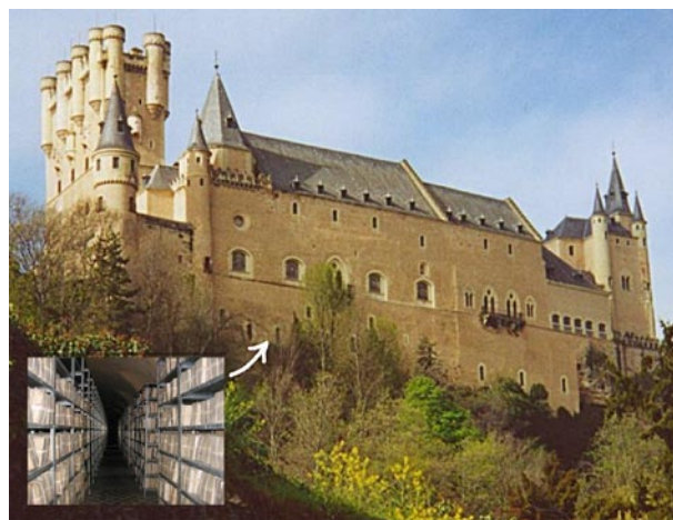
Figure 2. North facade of the Alcazar of Segovia, Spain. The narrow windows just visible over the shrubbery illuminate the military archive. The insert, bottom left, shows the interior of the archive.
