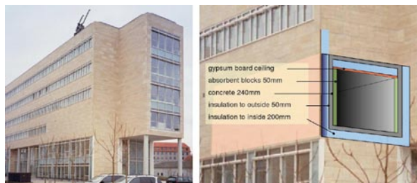
Figure 6. The building of Copenhagen University which houses the Arnamagnæan archive behind the windowless section of facade. On the right is a section through the archive. Note the thermal insulation against the interior of the building and the comparatively thin insulation of the outer wall. As a consequence, the archive temperature lies about midway between the outside temperature and the temperature of the core of the building.
