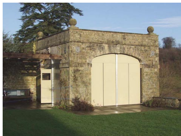
Figure 11. Detail of the construction of the enclosure
