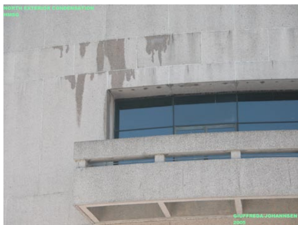
Figure 1. Condensed water leaking from the joints in the wall of the Smithsonian Institution’s Hirshhorn Museum and Sculpture Garden in the wintertime. (Photo by Gary Johannsen and Kevin Guifreda)
