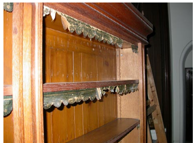
Figure 8. Damaged dust falls at Penrhyn Castle (National Trust), demonstrate the extent of cumulative abrasion that occurs between book spine and dust fall when books are removed from and returned to the shelves.
