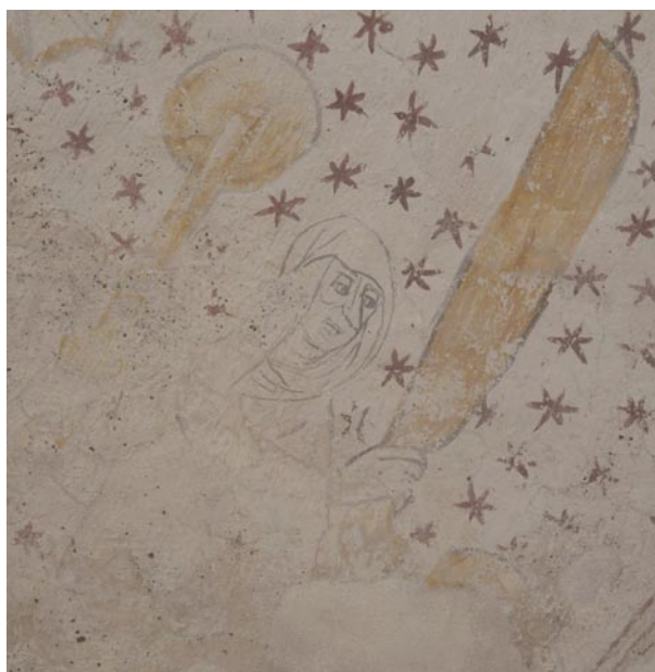
Figure 3. Detail of the wall paintings in Rorby church near Kalundborg. The paintings deteriorated by the precipitation of salts due to diurnal fluctuations in the relative humidity caused by intermittent heating. Photo by Roberto Fortuna, the National Museum of Denmark.
