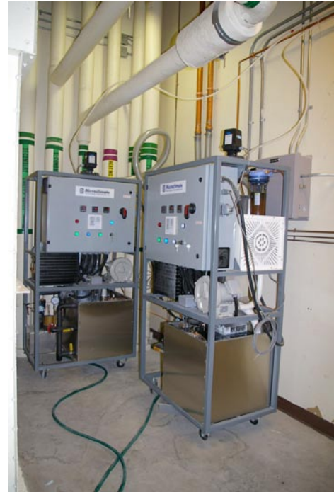
Figure 5. Two MCG 40s serving the Japan Gallery. On the closer machine can be seen the air filter (white grille), ion exchange cylinder and protective three-way valve (black unit on top of the machine)
