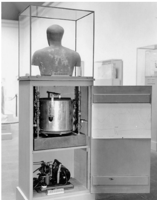
Figure 2. Electrically assisted passive humidity controlled display case, 1938
