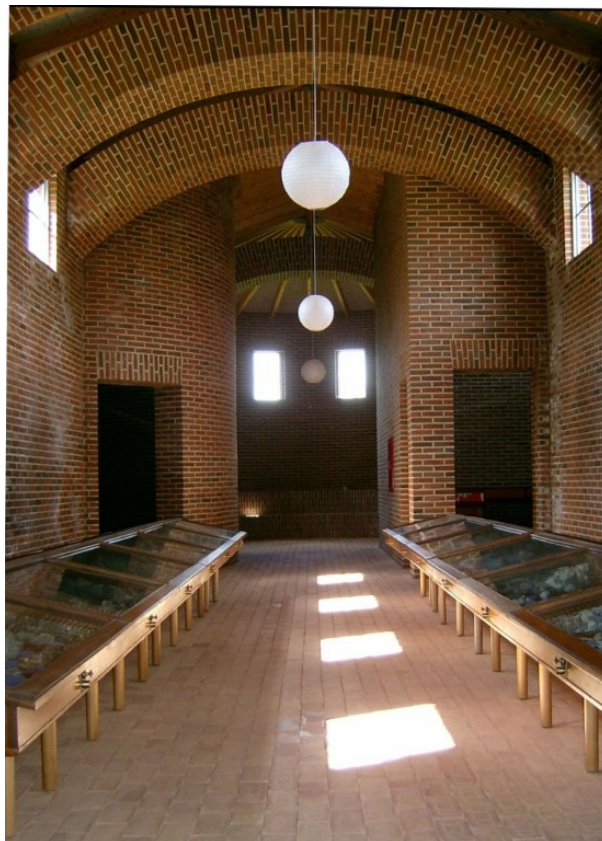
Figure 10: The Stone House has floor heating to a moderate temperature of 12-14 degrees. The warm floor provides thermal comfort for the visitors.
