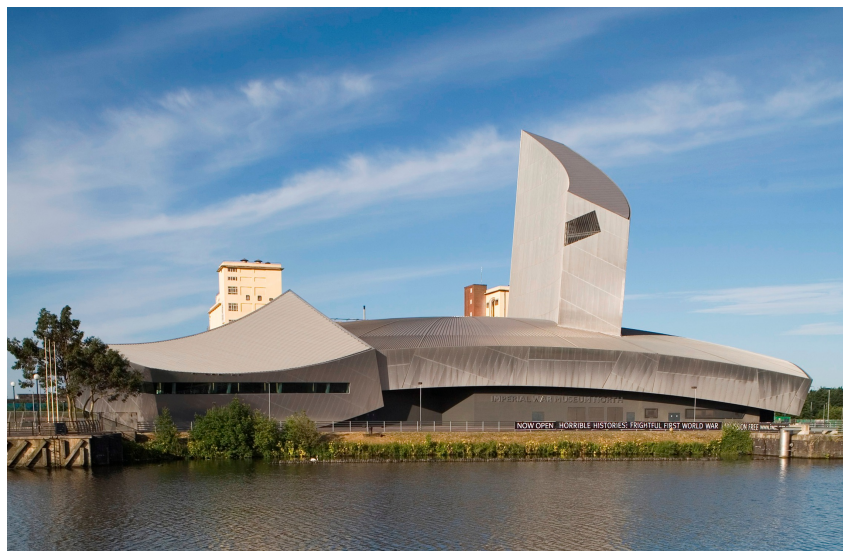
Figure 4: The exhibition building for the Imperial War Museum in Manchester, UK, is designed much like a submarine. The metal roof is a huge solar collector that heats up the space below in summer. (Courtesy of Imperial War Museum)
