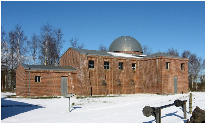
Figure 9: The 'Stone House' at Skærum Mølle was designed by the artist Per Kirkeby for a collection of minerals. The open land in the front of the building serves as a heat reservoir for the ground source heat pump.
