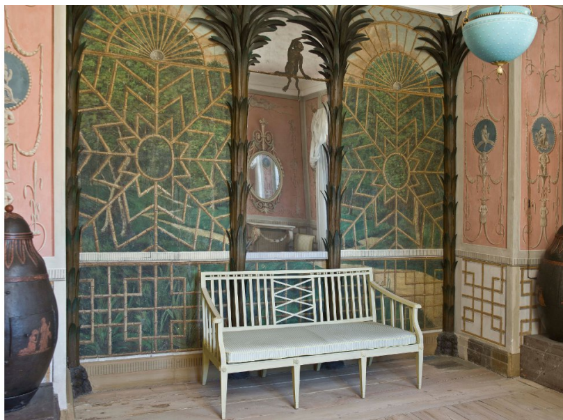
Figure 8: Interior view of the 'monkey room' in Liselund. The inlet of dry air is through the floor duct in the corner.
