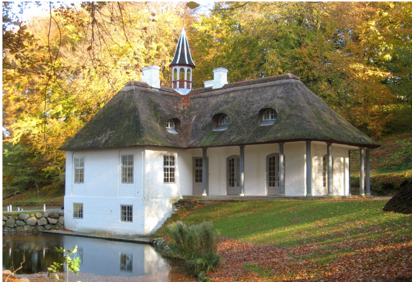
Figure 7: The country house in the romantic park Liselund has mechanical dehumidification all year to 60%RH. The temperature follows the outside running average.
