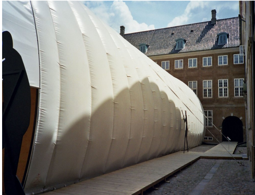
Figure 1: A temporary shelter for the exhibition of the Nydam Boat, an iron age warship, was designed as a pneumatic structure, located in a courtyard at the National Museum in Copenhagen.
