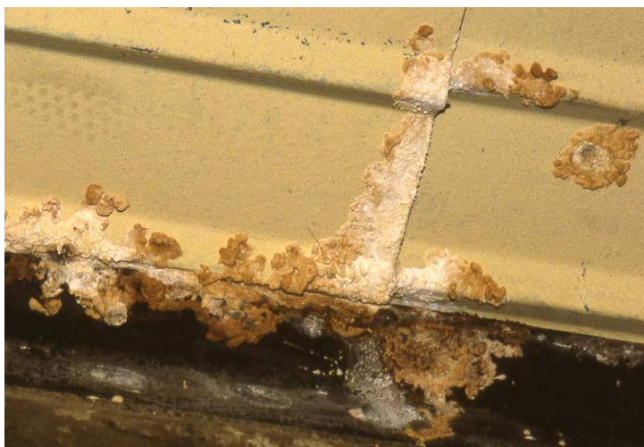
FIGURE 7. The ceiling of the Arts and Industries Museum is zinc coated steel. Condensation in the roof, aided by fireproofing chemicals, has corroded the zinc to white oxide, accompanied by fireproofing salts, ammonium dihydrogen phosphate, borax and a reaction product koktaite (hydrated ammonium calcium sulfate).
