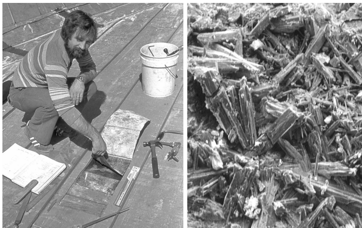
FIGURE 6. David Erhardt peels back a section of the one year old lead coated copper roof of the Arts and Industries Museum of the Smithsonian Institution. The lead was corroded by the damp plywood beneath it. On the right, a scanning electron micrograph (1mm across) of columnar crystals of cerussite, lead carbonate.
