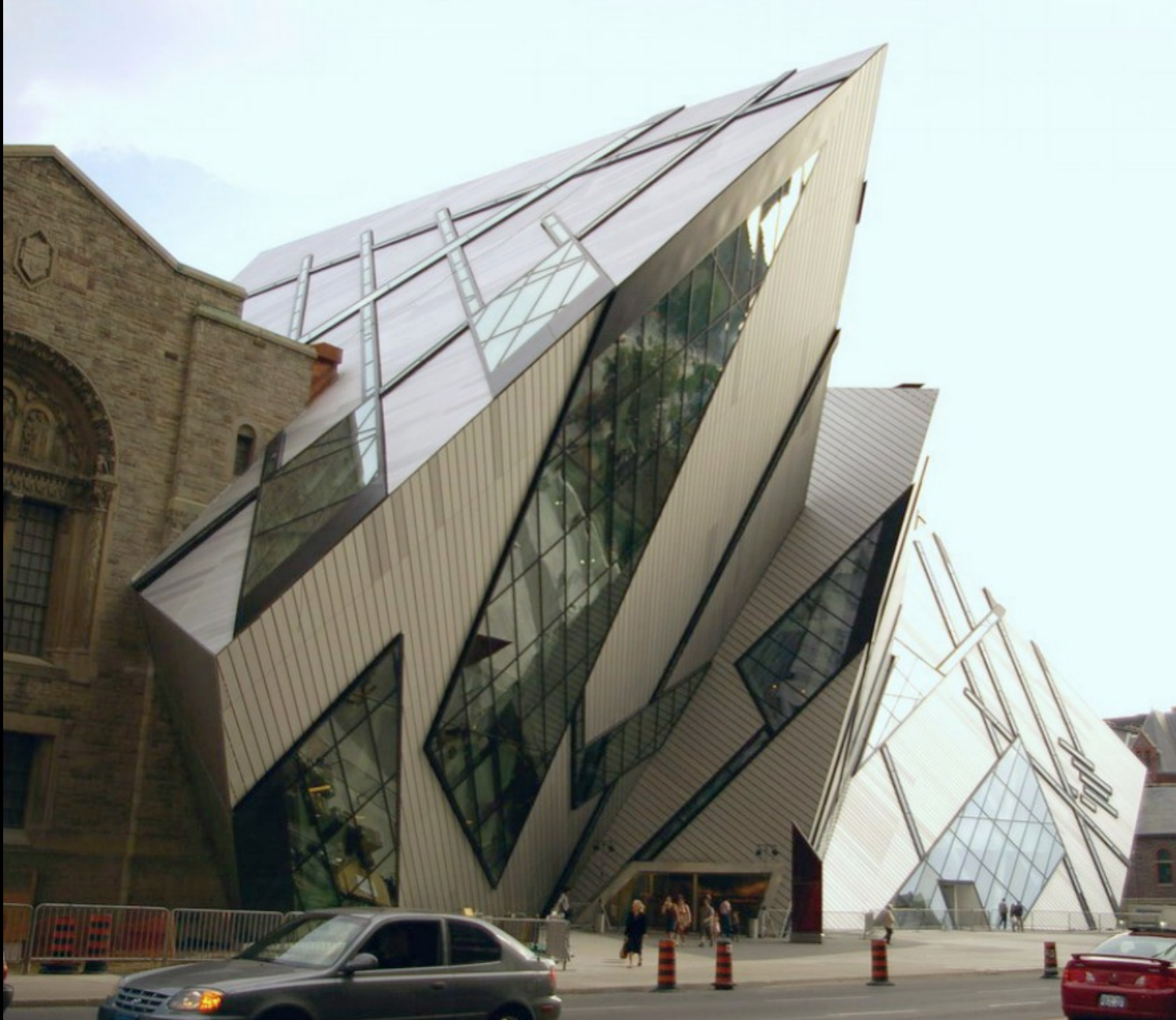
The Royal Ontario Museum, extension by Daniel Libeskind, 2007. Air conditioning of spaces was abandoned in favour of air conditioning of each showcase.
