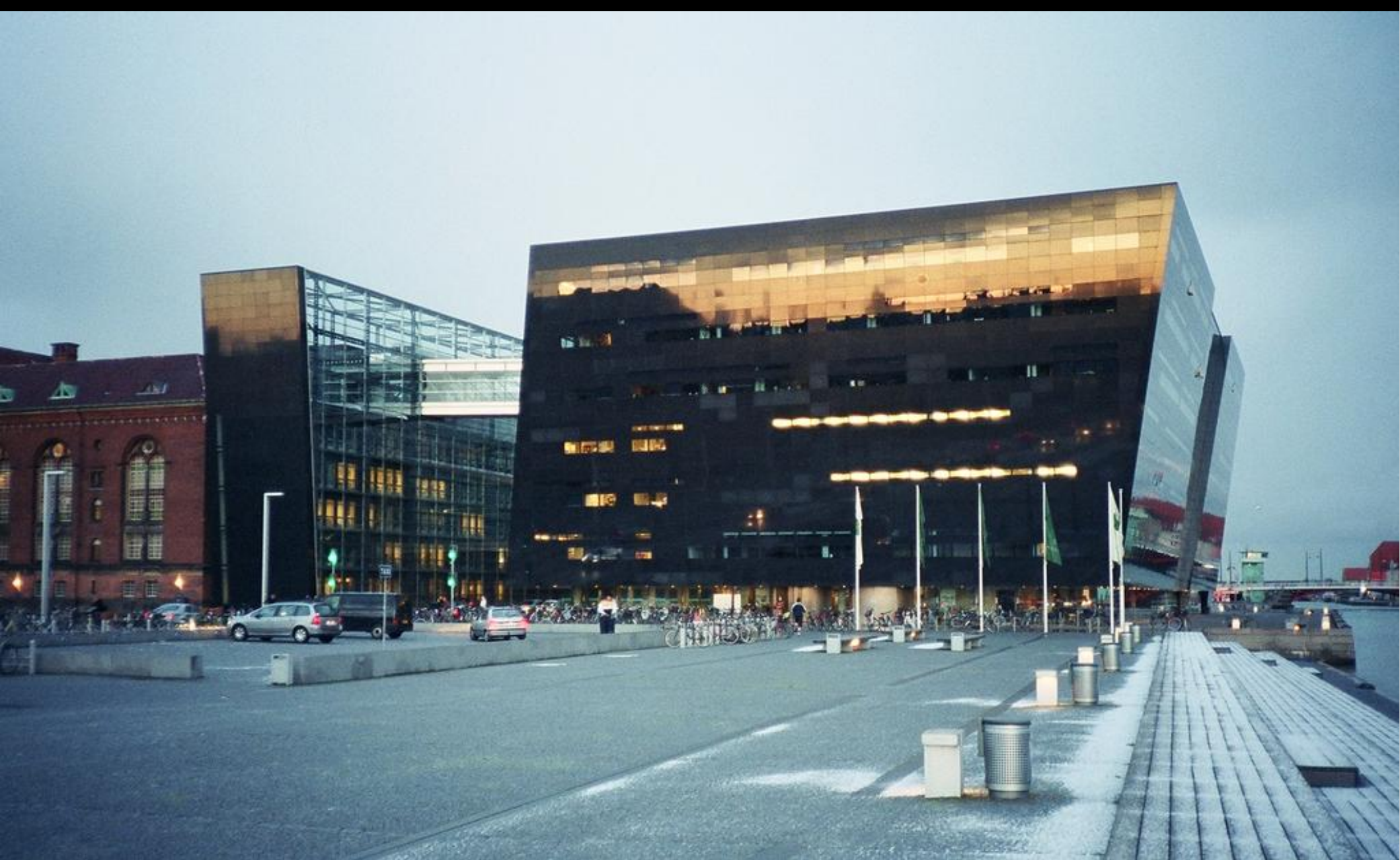
The Royal Library, Copenhagen. 1999. Architects Schmidt, Hammer and Lassen. An outward tilted wall cannot safely have high thermal capacity.
