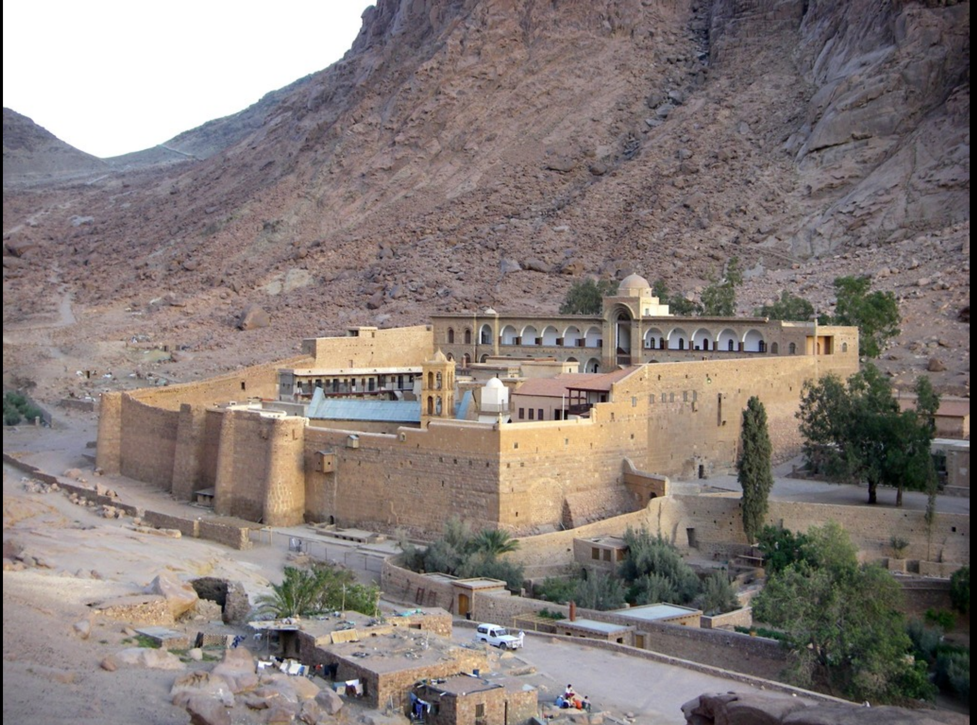
St. Catherine's Monastery, Sinai, Egypt
