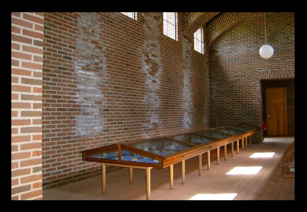
The white salt efflouressence shows where rainwater is leaking through.
