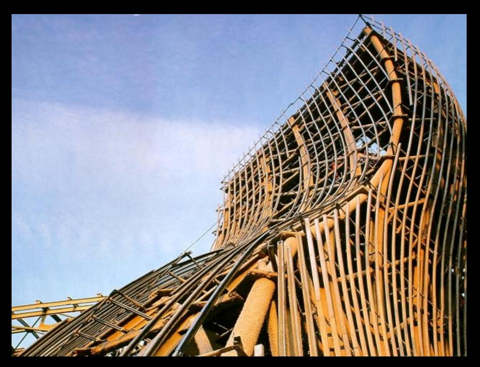
The steel framework forming the curved shapes of the building
