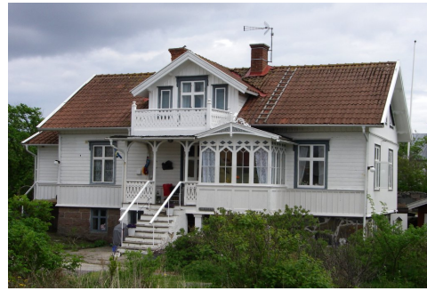
Figure 7: In the north, where it is nearly always too cool for human comfort, lightweight insulated structures are common. This house in Sweden is insulated with wood shavings.
