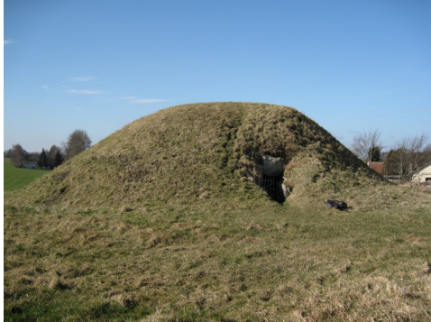
Figure 10: The grave chamber Maglehøj in Denmark. Built around 5000 years ago with a refined technique to keep the interior dry.
