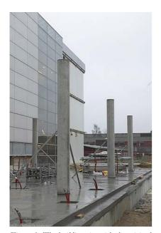
Figure 3. The building site with the original façade of block 1 and the additional constructions to support the new façade. (The Royal Library)
