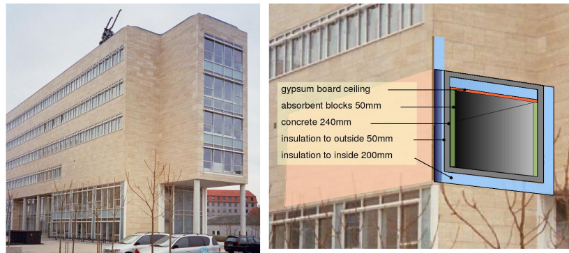
Figure 6: The building of Copenhagen University which houses the Arnemagnaeen archive behind the windowless section of facade. On the right is a section through the archive. Note the thermal insulation against the interior of the building and the comparatively thin insulation of the outer wall. As a consequence, the archive temperature lies about midway between the outside temperature and the temperature of the core of the building.
