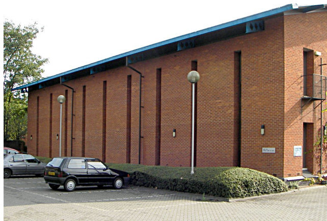
Figure 4: The Suffolk Record Office, Ipswich UK. The walls are 630mm thick, half of which is brick. It was built in 1990. The architect was Henk Piekma.
