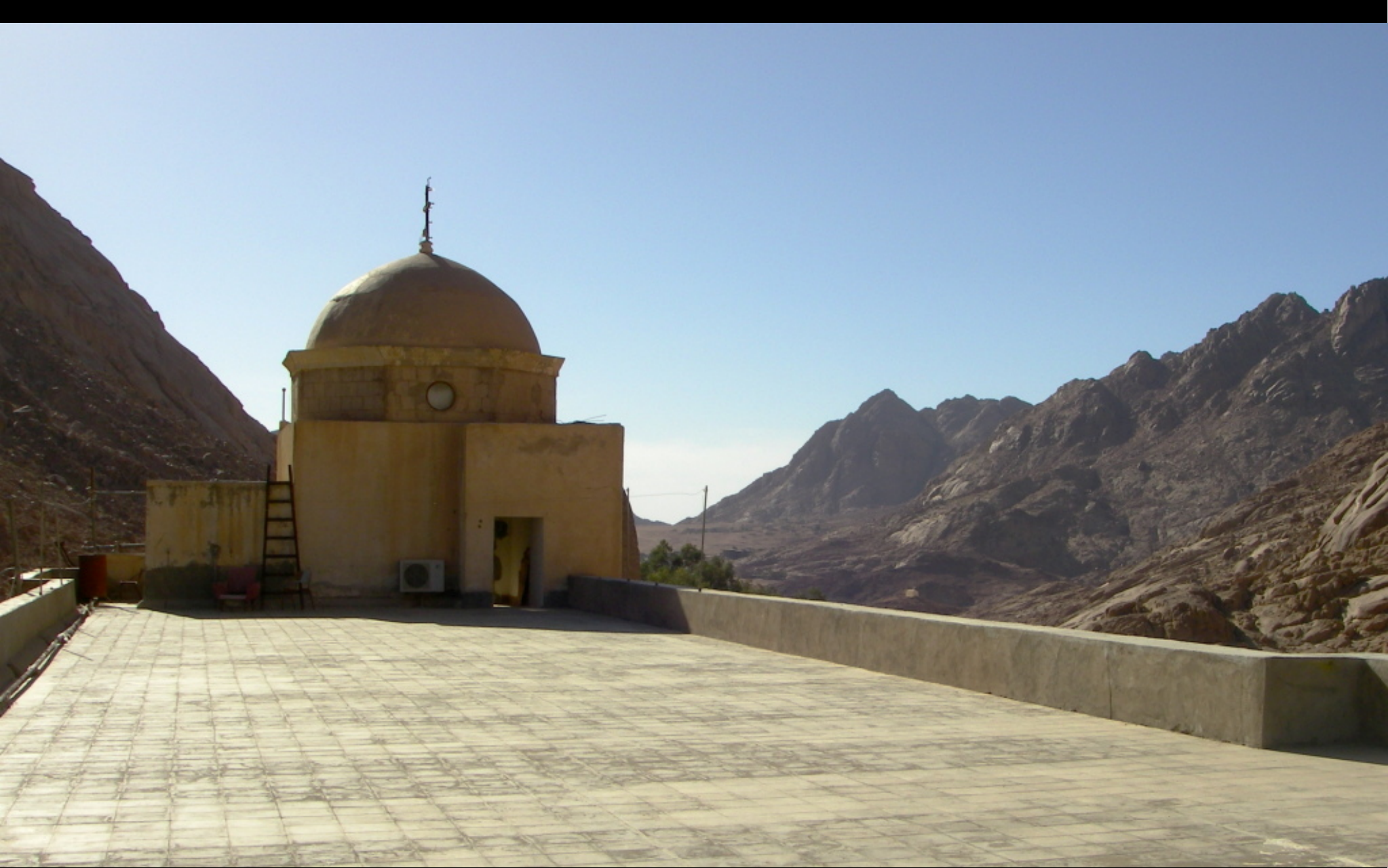
The library roof, looking west
