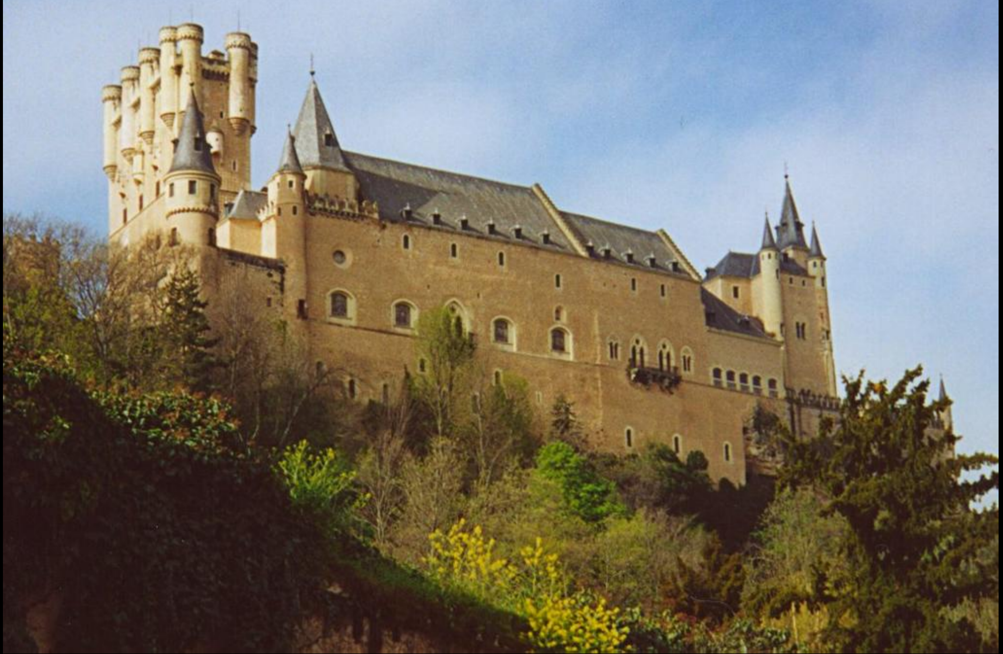
The Alcazar of Segovia, Spain. The military archive is behind the lowest range of small windows.
