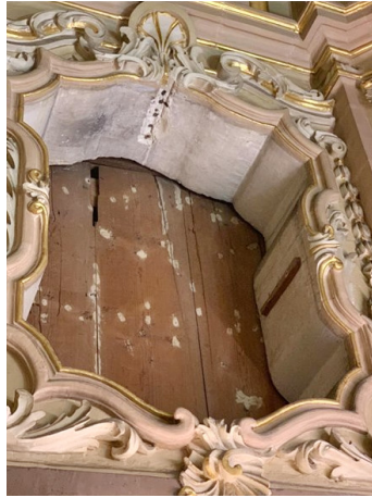
Figure 8: Wooden planks screening the stone wall behind a niche which usually holds a painting. Curia Church, Floriana, Malta. Photo by Valentina Lupo.
