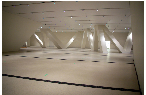
Figure 8. Garfield Weston Exhibit Hall, showing HVAC air supply grilles in the floor
