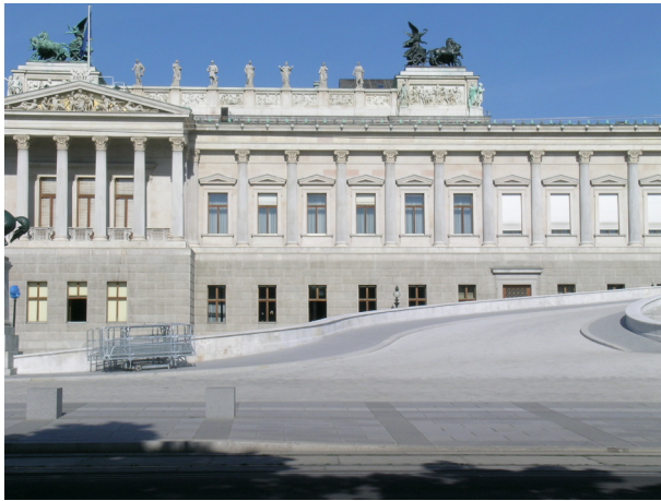
Figure 15. Twenty-six windows of the main facade of the Parliament are supplied with outer shading by means of plastic roller jalousies.
