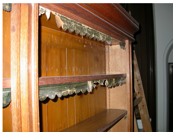
Figure 8. Damaged dust falls at Penrhyn Castle (National Trust), demonstrate the extent of cumulative abrasion that occurs between book spine and dust fall when books are removed from and returned to the shelves.
