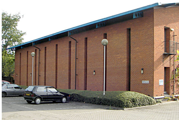
Figure 4. The Suffolk Record Office, Ipswich UK. The walls are 630mm thick, half of which is brick. It was built in 1990. The architect was Henk Piekema.
