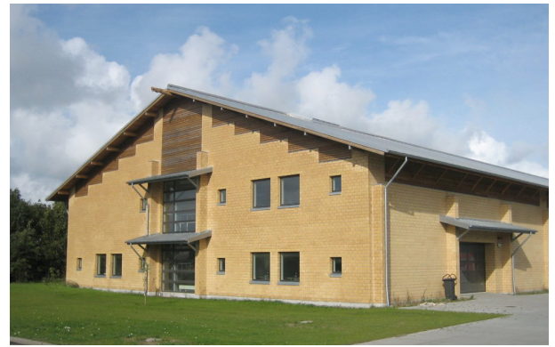
Figure 8. The recently constructed building in Ribe, providing storage for the regional museums of southern Denmark.
