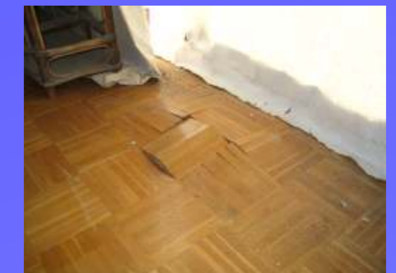
11. 12. The high level of RH, the architectural and design problems caused series of damages in the inner spaces of the Museum's new building.
