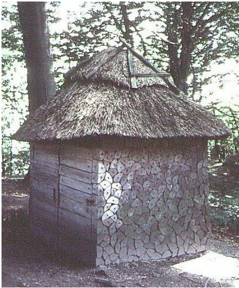
Figure 4.5 A small shed in the eighteenth century pleasure garden at Liselund on the Danish island of Møn. Sadly, the end-grain wooden wall is a sham: thin slices are nailed onto planks.
