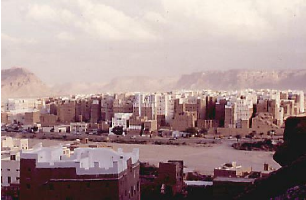
Figure 4.13 Panoramic view of Shibam in Yemen. Unbaked earth bricks are used to build up to eight storeys. Photo: Pia Olsen
