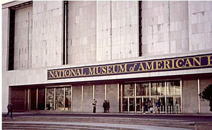
Figure 1.6 The National Museum of American History, in Washington D.C. On a bright spring morning the marble facade is stained by meltwater from ice that has condensed from the inside air.
