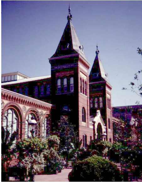
Figure 6.32 The Arts and Industries Museum of the Smithsonian Institution in Washington D.C. The south front showing the towers beside the entrance, used for cooling by the stack effect.
