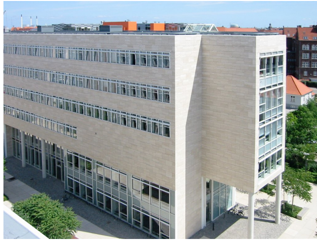
Figure 3: A building of Copenhagen University. The Arnamagnæan archive is behind the portion of wall without windows. It has no internal heating but gains heat from the core of the building, which is kept within the human comfort zone. Heat loss to the outside through thin insulation on the two exterior walls keeps the archive temperature about midway between indoor and outdoor temperatures.
