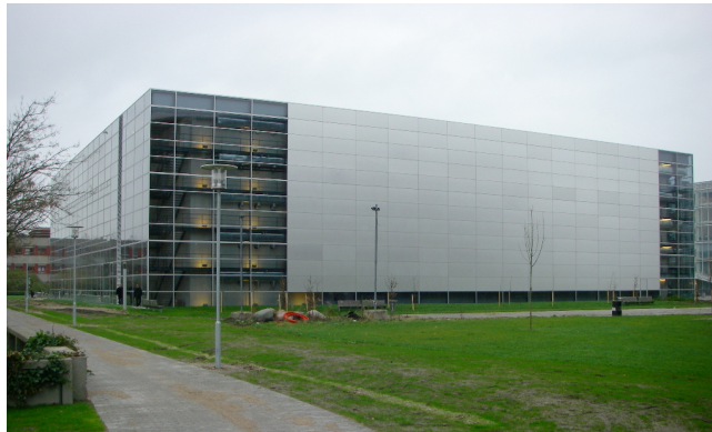
Figure 1: A storage building of the Royal Library in Copenhagen, completed in 2000. It is permanently air-conditioned to a set point at 18°C and 50% RH.
