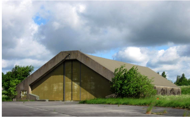
Figure 3: A fighter jet shelter from the cold war, at Værløse, north of Copenhagen. The reinforced concrete shell is 600 mm thick. It is now used as a furniture store, mechanically dehumidified to 50% RH.
