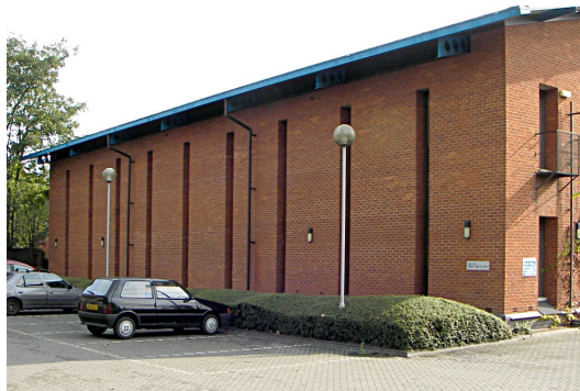
Figure 11: The Suffolk Record Office, Ipswich, UK. It was built to work with only winter heating to control the climate. The walls are both massive and thermally insulated.
