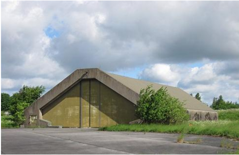
Fig. 9.2. Shelter 209 storage building.
