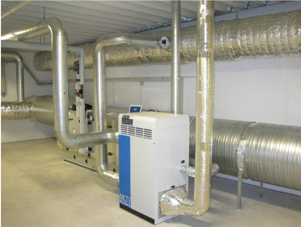
Fig. 4.15. This one desiccant dehumidifier controls the entire basic climate storage area in Vejle (approximately 17,000 m 3 ). Model: Munters MLT 800, max. power consumption at full load 5.12 kW, nominal airflow 800 m 3 /hour, approximate dehumidification capacity for maintaining 50% RH at 12 °C: 2.8 kg/hour (data from Munters product information).
