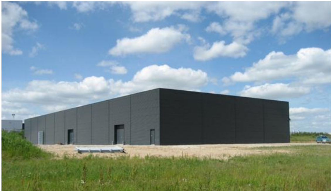
Fig. 5.1. The storage facility in Randers.
