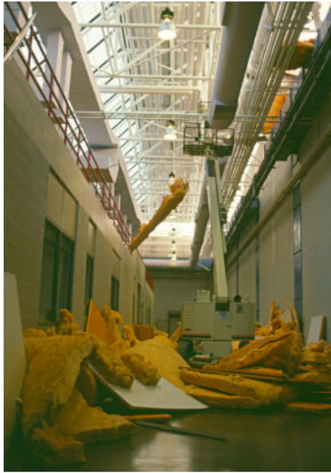
FIGURE 20. Ceiling insulation being stripped from a museum store in Maryland, USA, because of condensation on the roof above. Condensation only occurred on the half of the long 'street' that was badly sealed.
