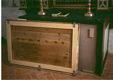
FIGURE 4. The back of the new frame supporting the old picture, at the time of installation. The new timber was attacked by mould within one year, though the original oak planks were unaffected.
