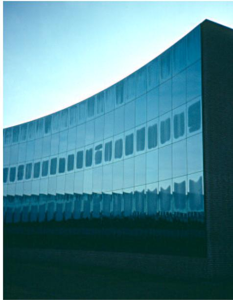
FIGURE 19. The north east facing facade of the IBM building in Lundtofte, near Copenhagen, photographed on a cool evening. There is condensation on alternate levels of the glass facade, which shows as dark patches, in contrast to the clear reflection of the sky in the unaffected glass. An apparently homogeneous facade has systematically uneven hygrothermal characteristics.
