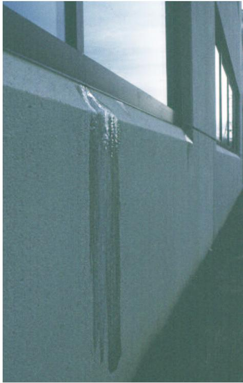
FIGURE 22. Ice accumulating from water vapour leaking through a gap in the air barrier of the museum store in Maryland.
