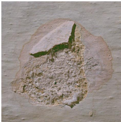
FIGURE 2. Pink discolouration of biological origin, probably a halobacterium, around an efflorescence of salt on the inner side of the wall of Gierslev Church, Sealand, Denmark. The picture is about 15 cm across. Photo by Roberto Fortuna.
