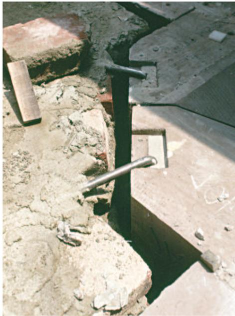
FIGURE 28. The 1 inch (2.5 cm) gap established between the brick structure and the new stone (actually coloured concrete) decorative elements. Sensors were placed in this gap and at other places in three sections through the building.
