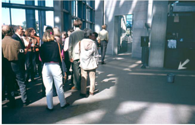
FIGURE 18. The bucket (arrowed) catches dripping condensation from the skylight. The National Gallery of Art, Ottawa
